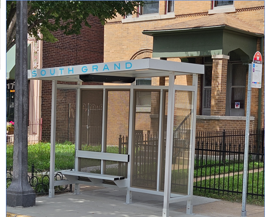
MetroBus shelter with perforated metal walls, allowing for transparency and easier maintenance
