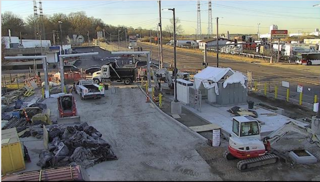
North Broadway Transit Center E-bus En-route Charging Infrastructure
