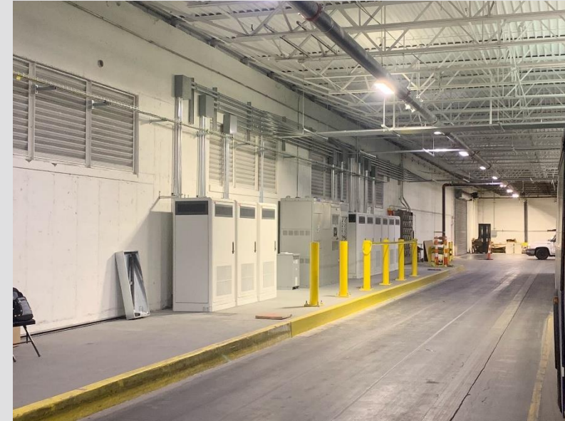
Brentwood Bus Facility E-bus Charging Infrastructure
