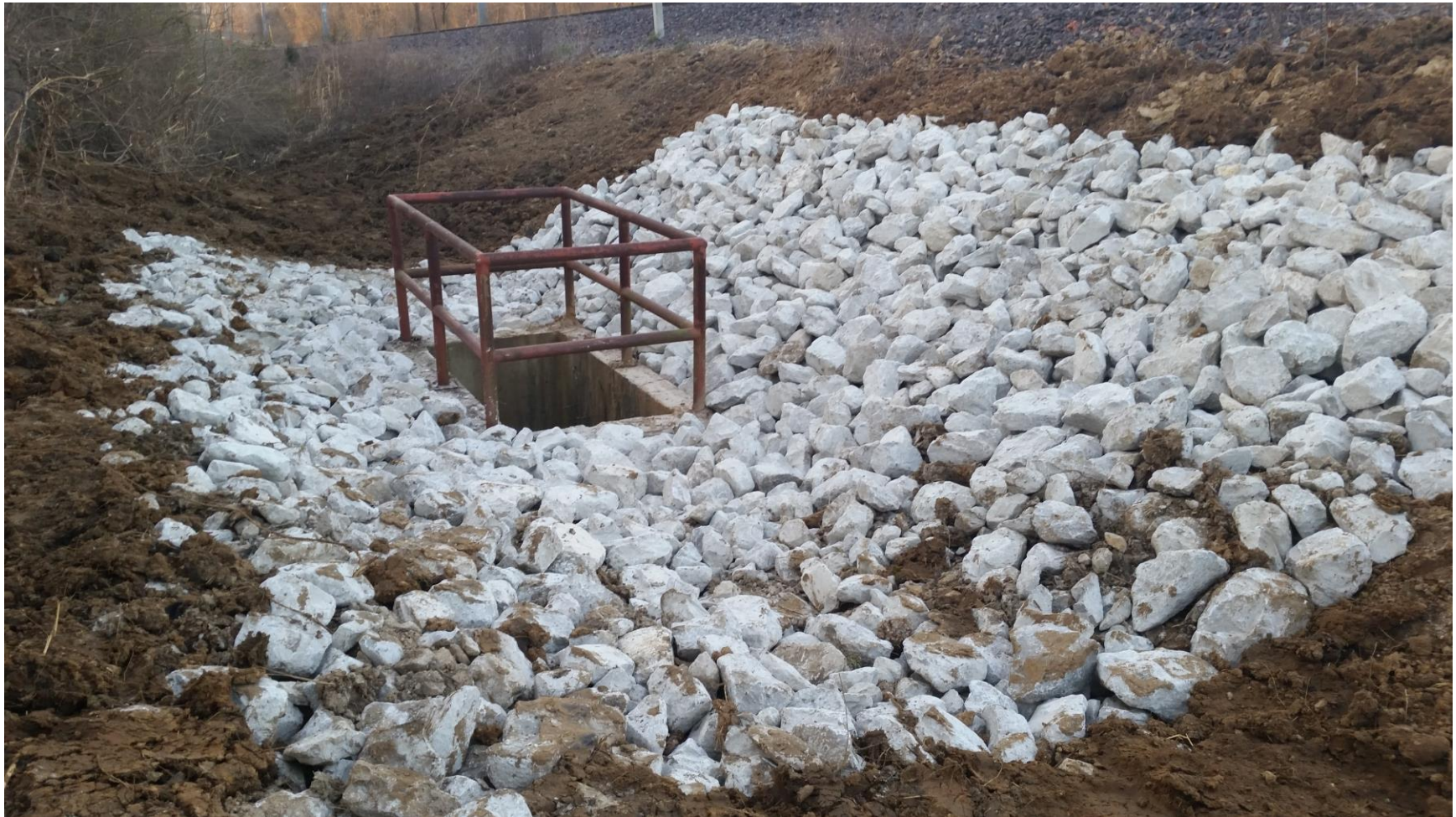
Bank Stabilization and Scour Protection at Drainage Structure Inlet
