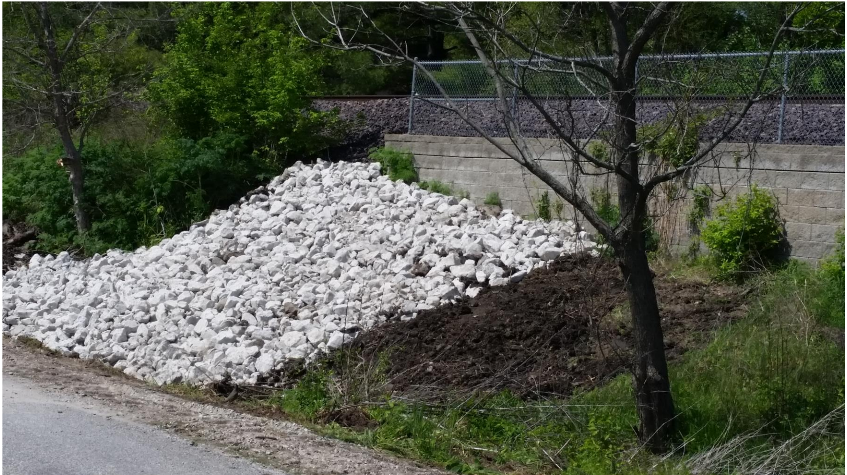
Slope stabilization and buttressing adjacent to a MetroLink retaining wall.
