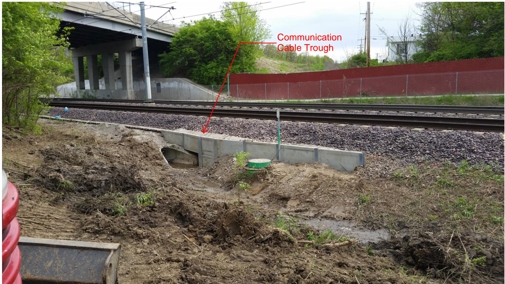
Installation of a Ballast Retainer structure adjacent to a culvert outlet. Scour from the culvert had led to undermining of the Communication Cable trough running parallel to the alignment.
