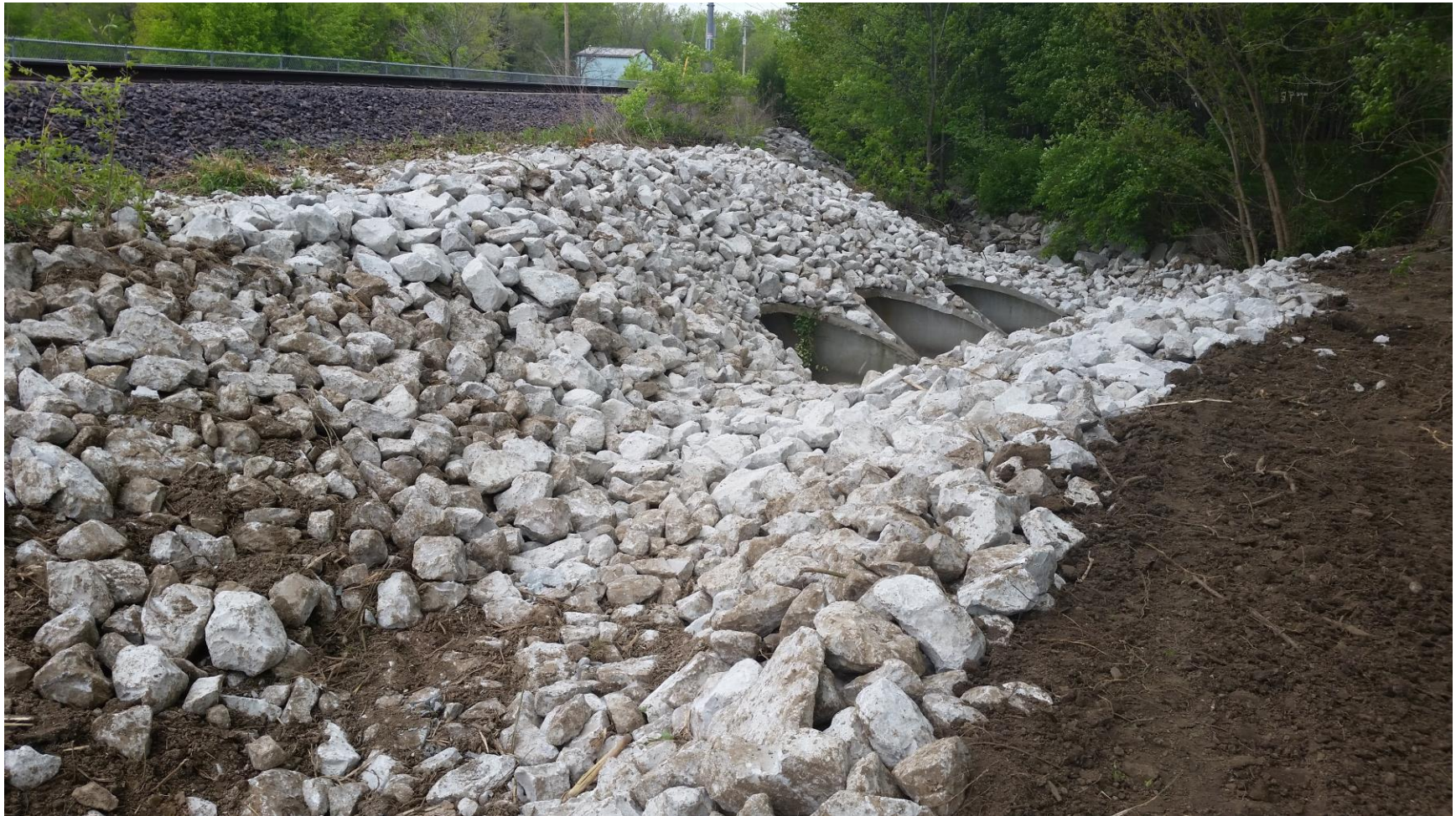
Installation of scour protection and bank stabilization at a triple culvert outlet.
